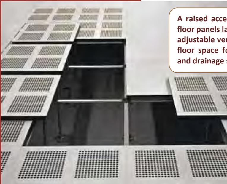
A raised access floor comprises of load bearing floor panels laid in a horizontal grid supported by adjustable vertical pedestals to provide an under floor space for the housing of electrical cables and drainage systems
